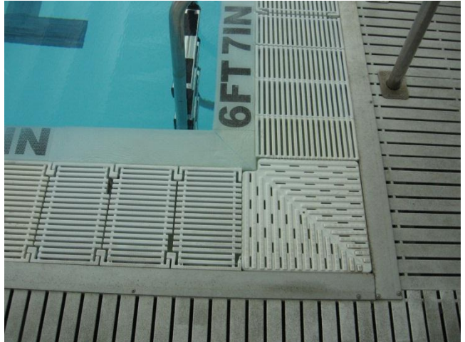
Gutter overflow system
