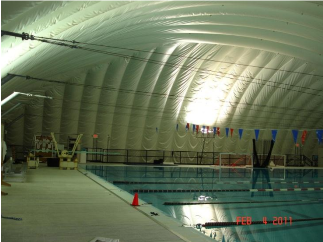
Interior Pool View #3
