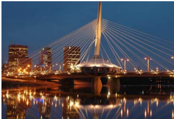
The Provencher Bridge in Winnipeg - Photo by Richard Marquez
